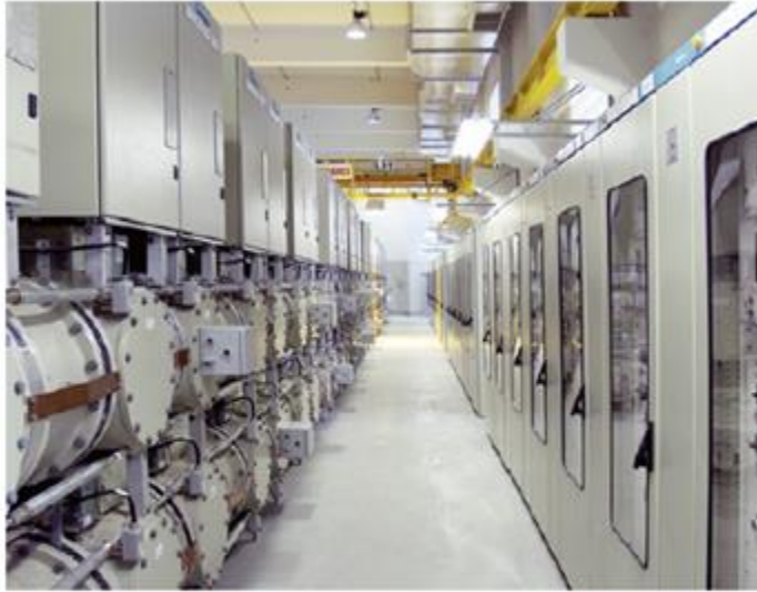
GIS for a rated voltage of 145 kV AutomationForum.Co
